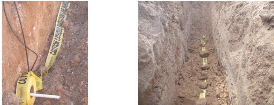
Figure 30. Installation of warning tape in a cable trench.
