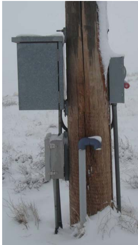
Figure 50. Installed impressed current system showing rectifier, anode junction box, external circuit breaker switch, and vent pipe.
